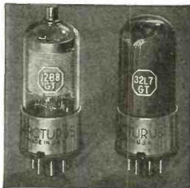
available. Tube Type 32L7GT, for instance, may be used in conventional half-wave high-vacuum rectifier and beam power amplifier circuits. Type 12B8GT has both a pentode and triode section, the former being used as a conventional R.F. or I.F. amplifier and the latter as a biased or grid-leak detector. Neither tube is any larger in size than the conventional GT Midget tubes.
