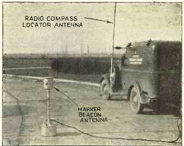
Mobile type of short-wave guide-beacon station.
