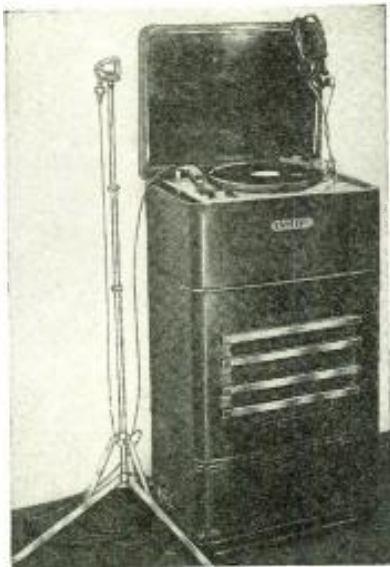
Console type recorder, with folding "mike" stand and headphone monitor.
