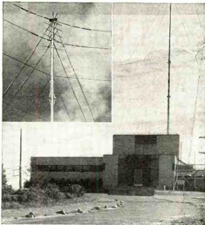
Photo at left shows Harry Whitmore at the transmitter panel of WIXOJ, frequency modulated station at Paxton, Mass. Photos at right show transmitter building at Paxton; 50 kw. equipment under construction. Insert shows transmitter antenna mast, with 4 bay turnstile aerials and vertical aerial on the peak.
