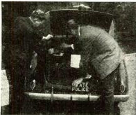
F.M. police equipment installed in luggage compartment of radio car.
