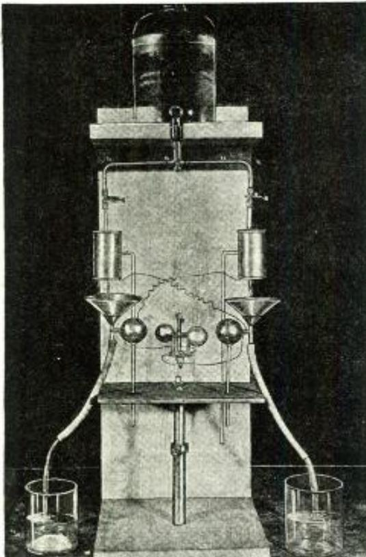
Left: The remarkable apparatus all set up—the electric charge accumulated from dropping water operates a motor.
