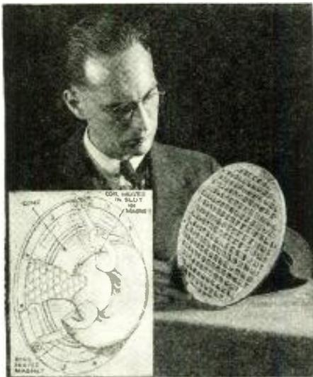
The new loud speaker—and a diagram showing its construction.
