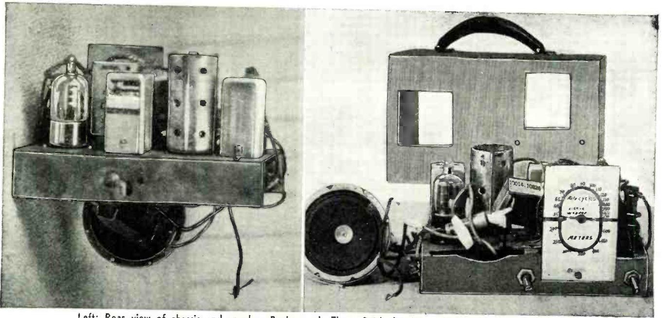
Left: Rear view of chassis and speaker. Background: The unfinished cabinet. Right: Front view of chassis.
