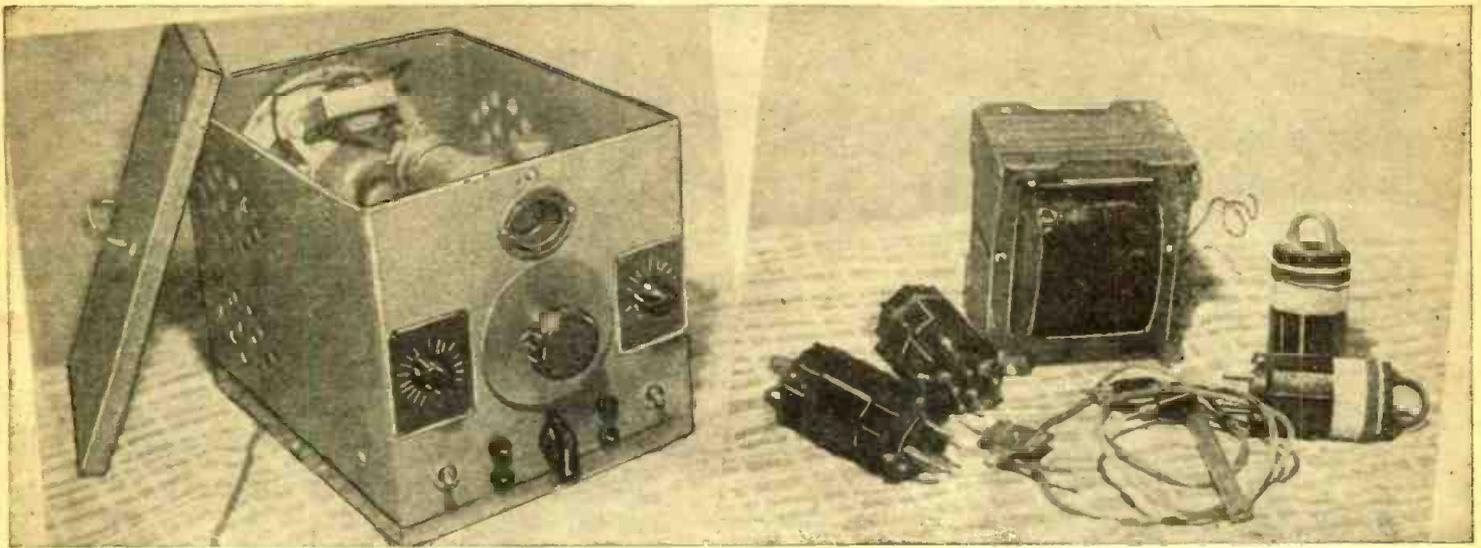
Photo at left shows general view of the "signal-tracer," while the photo at right shows the parts used in building it.
