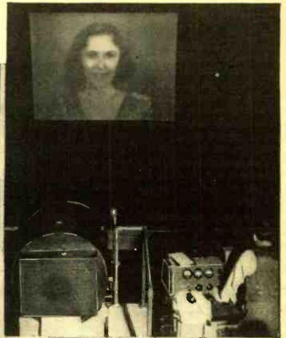
Left: An engineer inserts the high-voltage kenetron in the theater projector. Above: View from theater balcony, showing projector, and image on screen.
