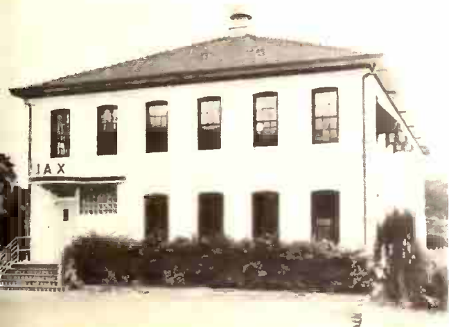
City Owned Headquarters
