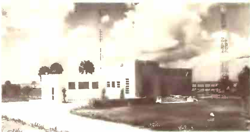
Modern Transmitter House
