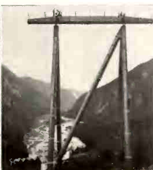
AVALANCHE-resistant pylons carry power for famed aluminum smelter at Kitimat
