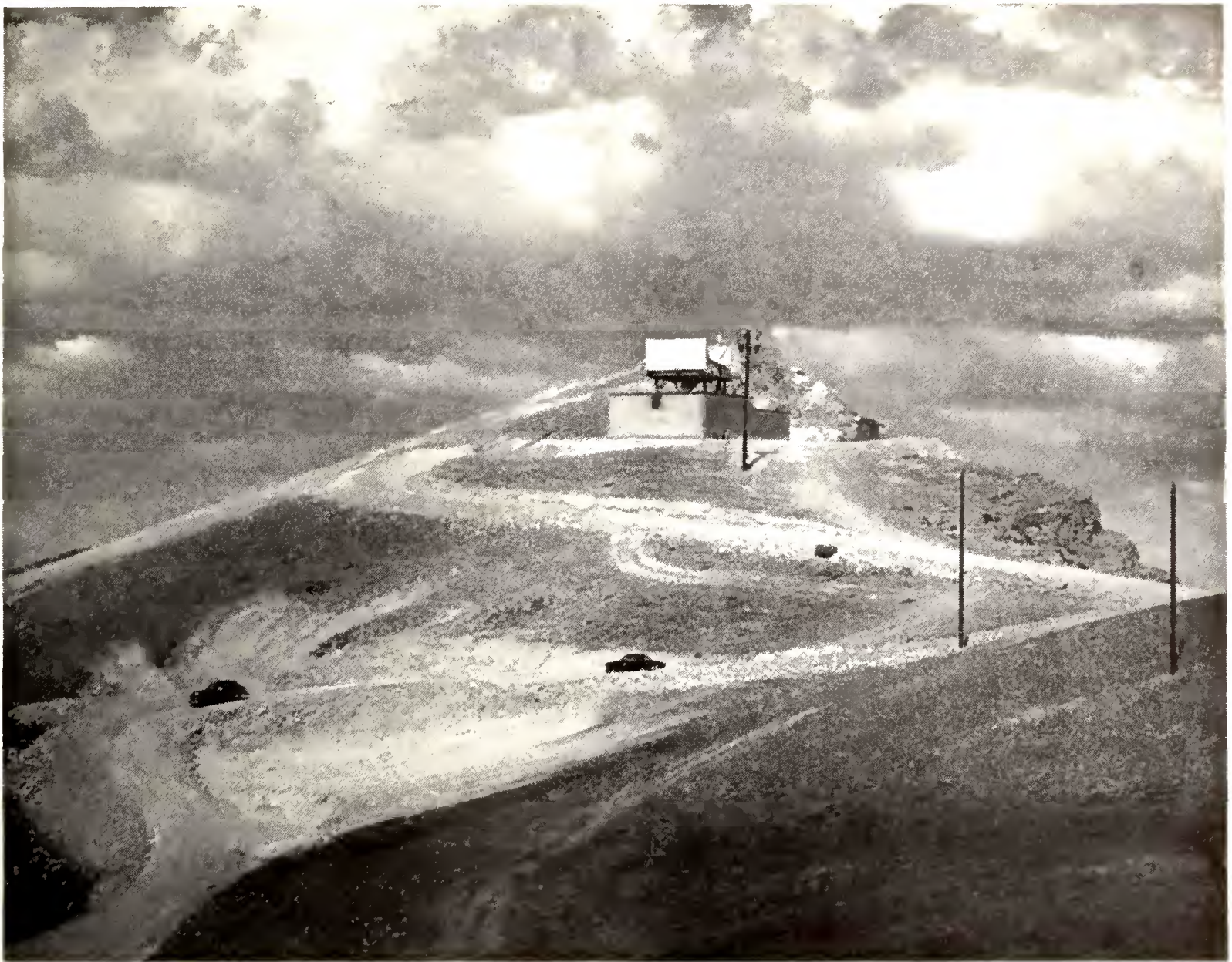
Access road to radio relay station, Rocky Point, Nevada.
