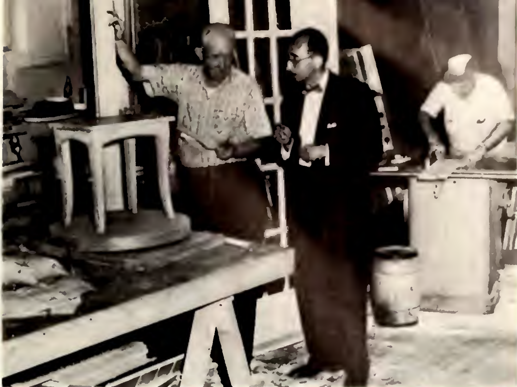
1. Set: Greatest saving in producing several commercials as a unit comes through set construction and labor. Above, Robert Lawrence Productions carpenter shop
