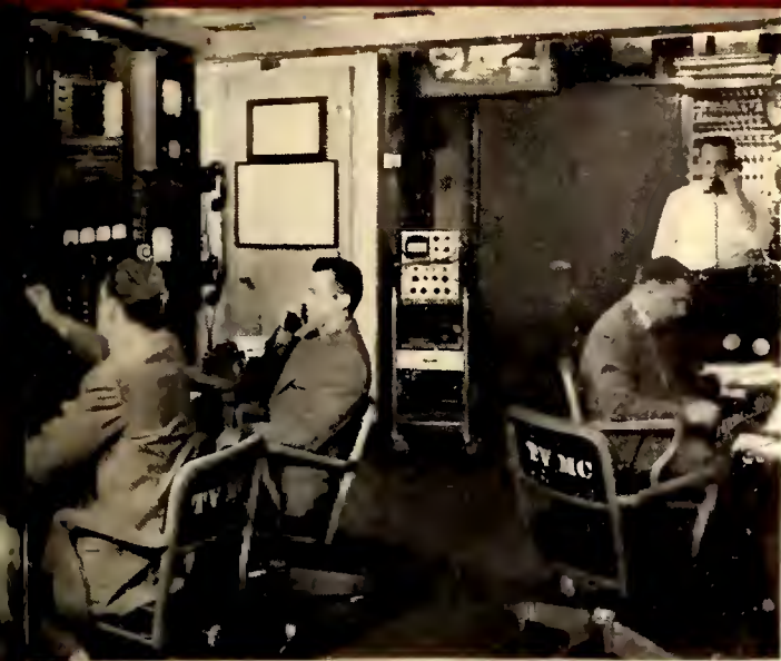
NERVE CENTER of ABC-TV operations—the master control room—is largely RCA equipped.
