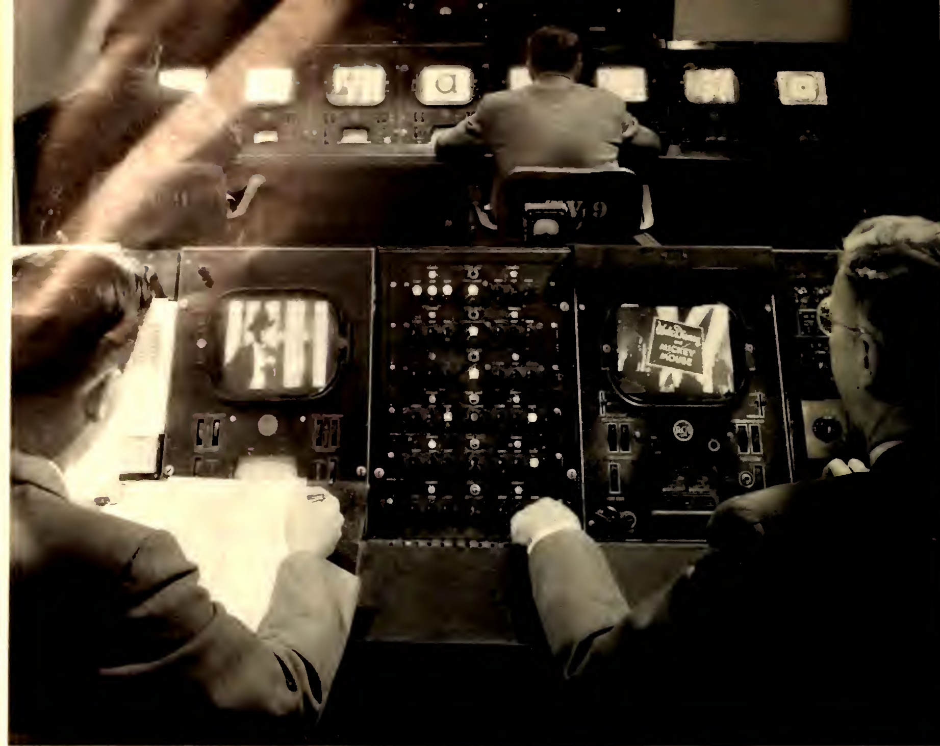
"FILM CENTRAL" for network operations. From this control room all the ABC film shows are fed to affiliates.
