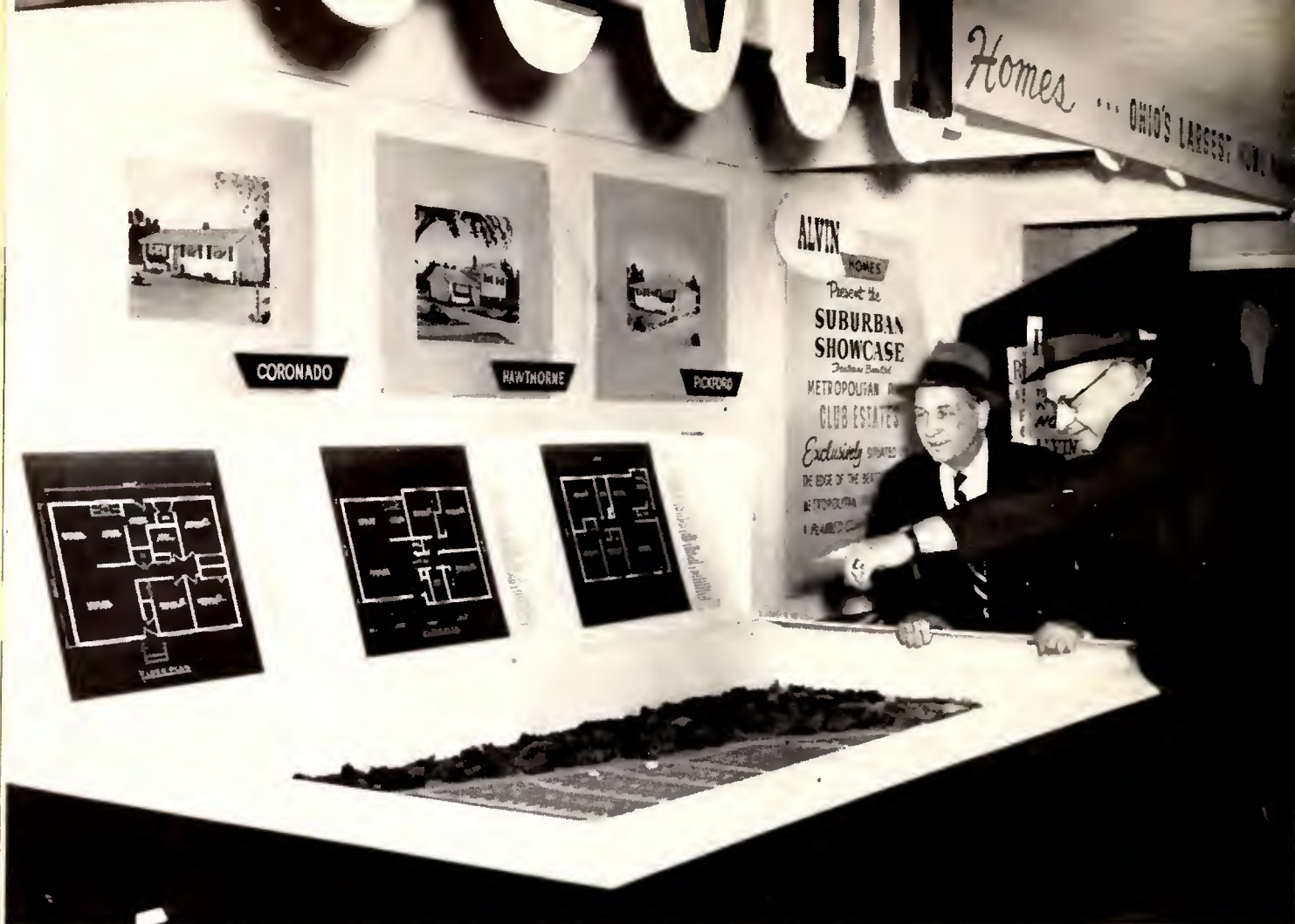
CLEVELAND builder Al Mars, president of Alvin Homes there, points out features of a plot display to John Cameron Swayze, m.c. of ABC Radio's daily weather show sponsored by Lennox. Swayze's in town to plug Alvin as part of package offered for installing Lennox heating systems.
