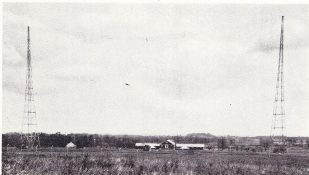
General view of the Whippany Station, 3XN
