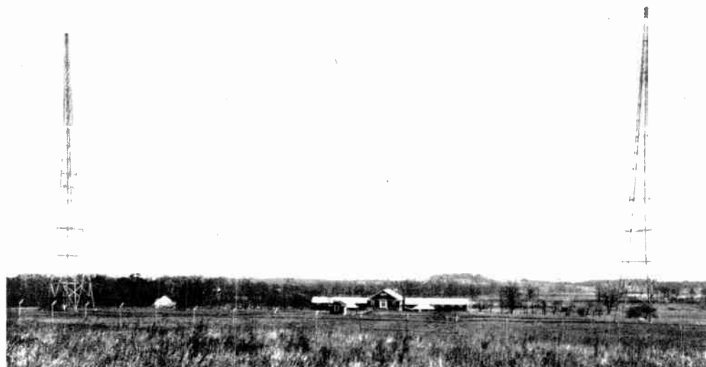
General view of the Whippany Station, 3XN
