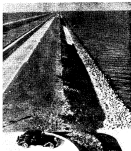
The great dyke, built to allow drainage of the Zuider Zee (Ijssel Lake) to create new farmlands. The narrow strip of concrete on left is a bicycle path.
