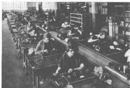
Synchrophase Wiring Assembly
