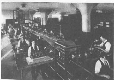
Final Inspection and Testing
