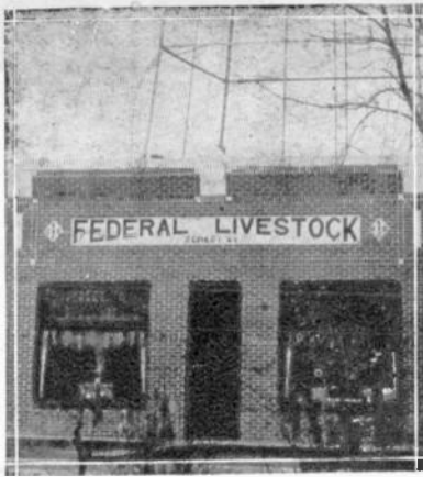
EXTERIOR VIEW STATION K-G-B-Z
