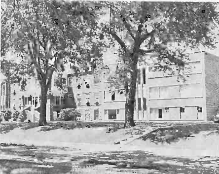
The Falls City Community Hospital has a 42 bed capacity and 8 bassinets; this includes the new 14-bed additional wing recently built.
