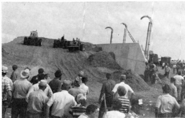
Farm Director Cliff Adams watched as this new concrete bunker type horizontal silage storage structure was filled with corn silage.
