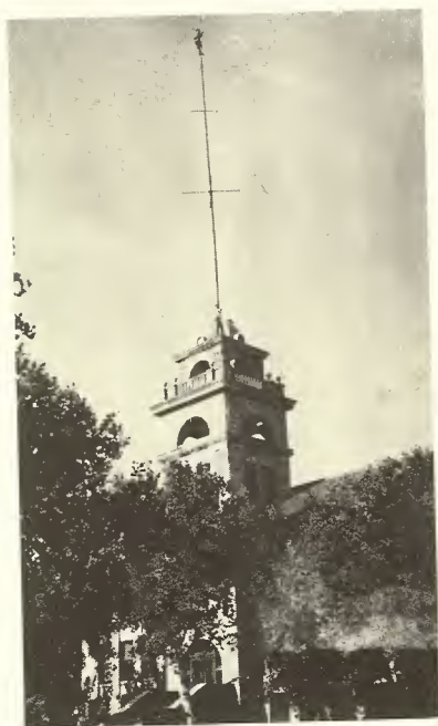
Dean Goddard standing on the tower of the Engineering Building to assist Robert W. Stewart (at top of mast) in attaching supporting cables to the 120-foot aerial. (R. W. Stewart photo)
