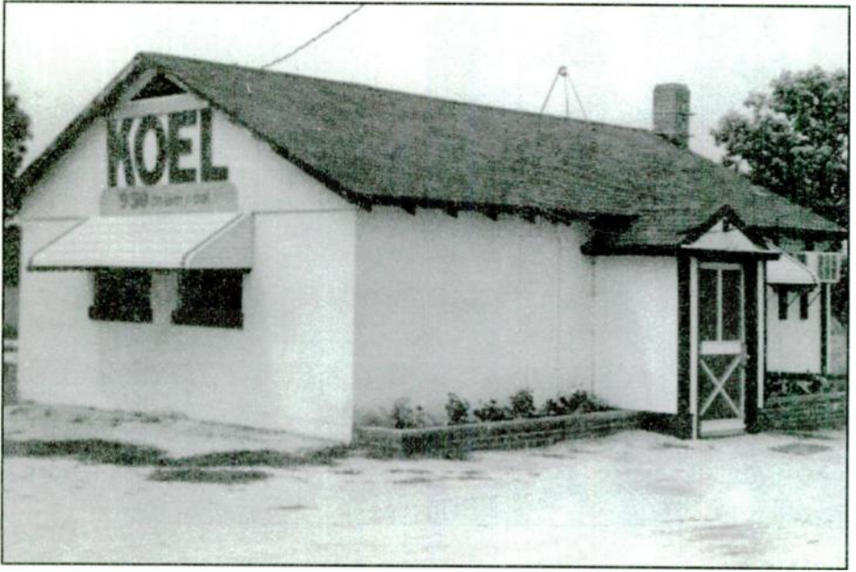
KOEL - AM transmitter facilities located on the east edge of Oelwein.
