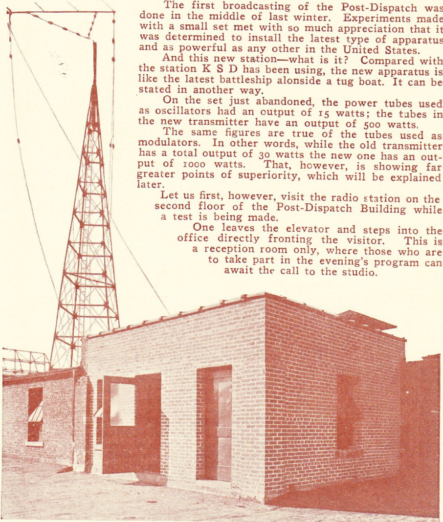
Brick structure on the roof of the Post-Dispatch Building erected to house the transmission apparatus, motor generators, etc. The studio is on the second floor. Metal conduits to the roof are grounded every few feet to prevent the possibility of picking up strays.
