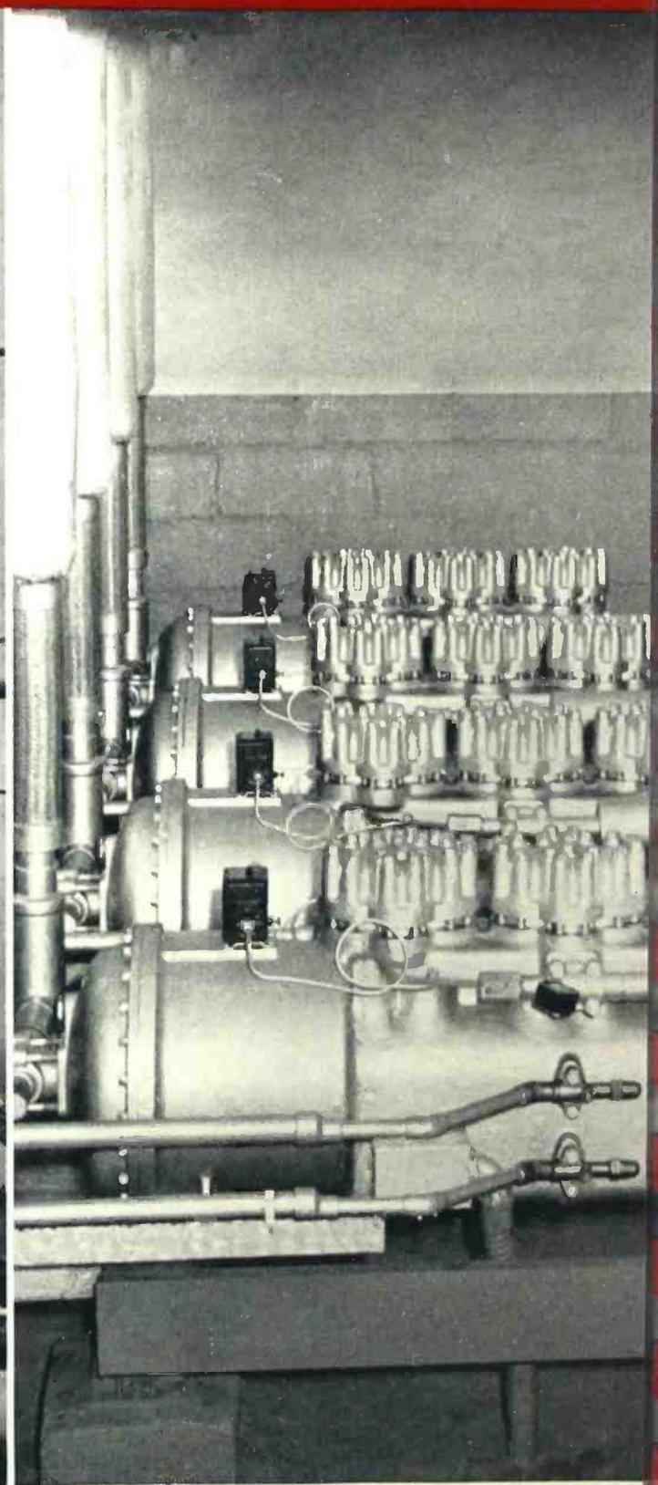
All KYW studios and offices are completely air-conditioned with equipment manufactured by Westinghouse Air Conditioning Division. Four 25-ton condensing units are operated in a series. 200 gallons of water a minute are required for the four machines. Three evaporating condenser units on the roof aerate the water and reduce its temperature so that it may
