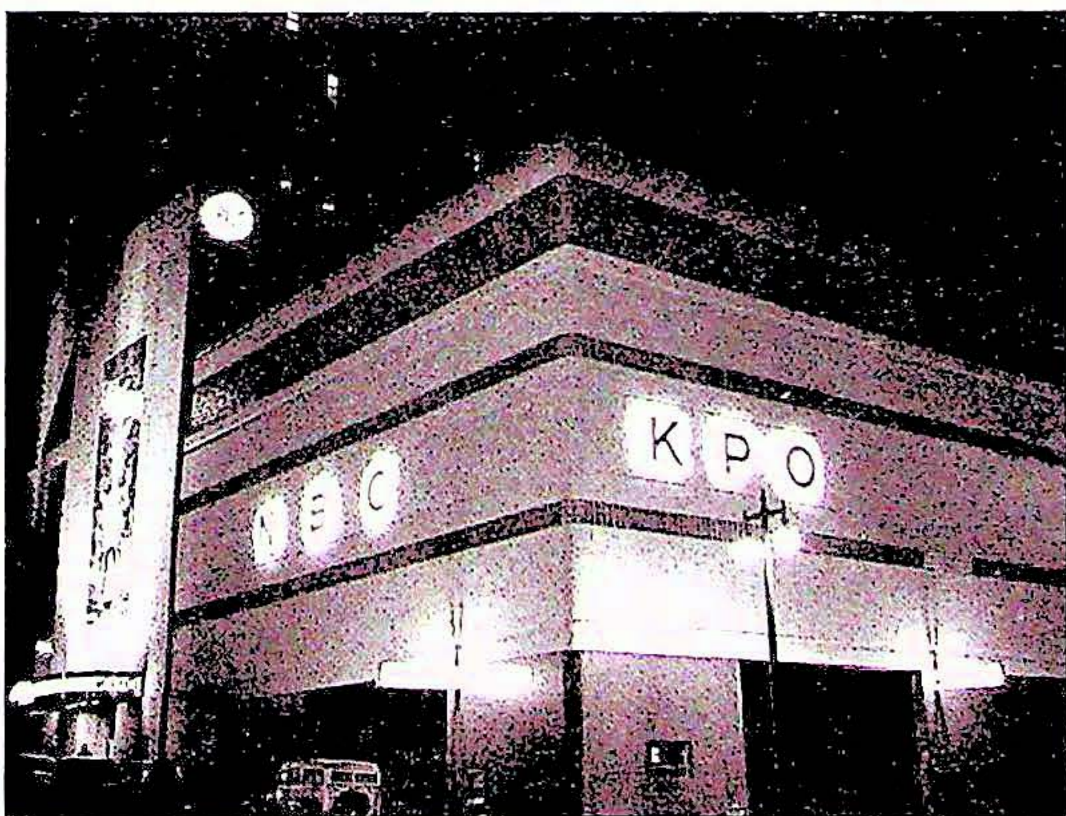
View of NBC-KPO studio and office building, San Francisco.
