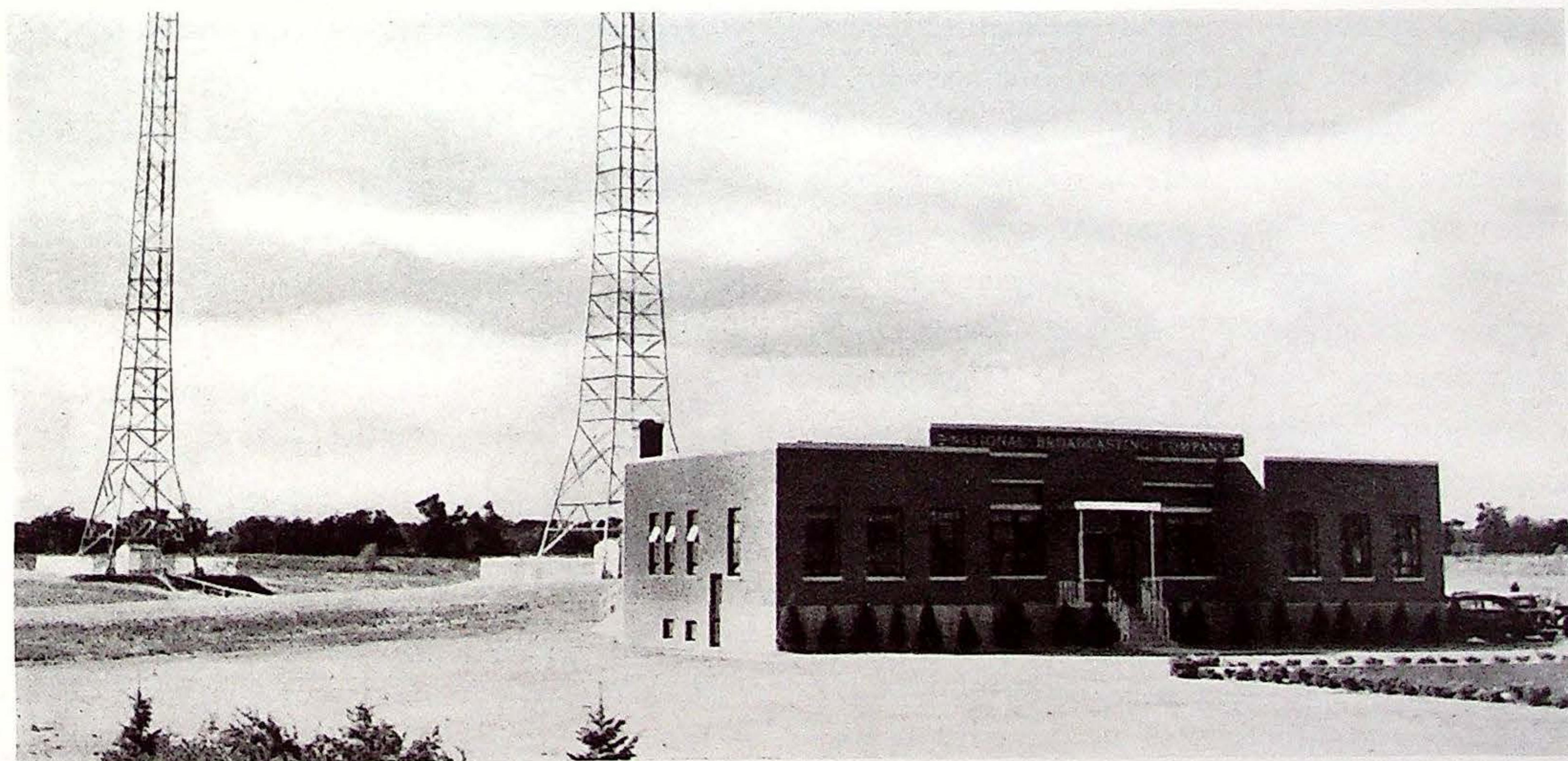
Transmitter building and vertical radiators of WNBC at Port Washington, L. I. 50,000 watt key-station of NBC in New York.
