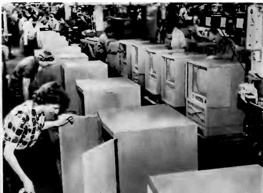
Cabinets under final inspection on RCA Victor's TV assembly lines.
