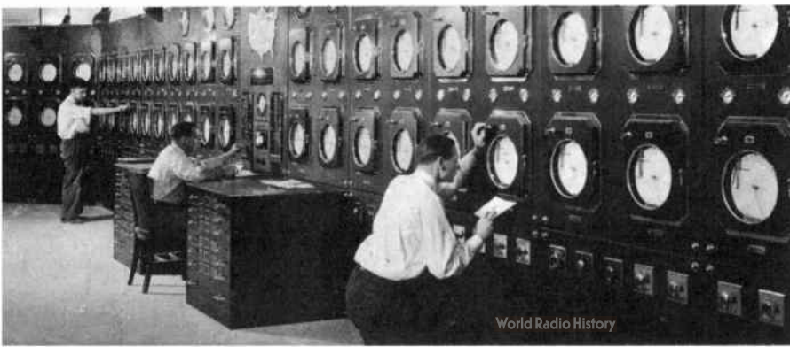
Above: Master control desk, nerve center of broadcasting in the RCA Building, designed and built by RCA Engineers. Left: Control board of the studio air conditioning plant.
