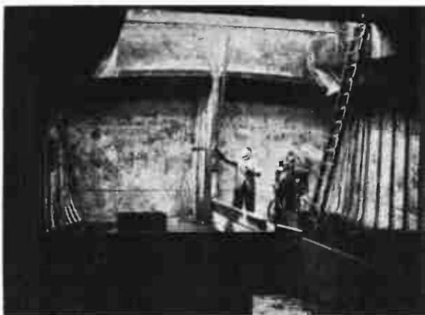
*The hold is prepared for the addition of 200 tons of concrete as ballast.*
