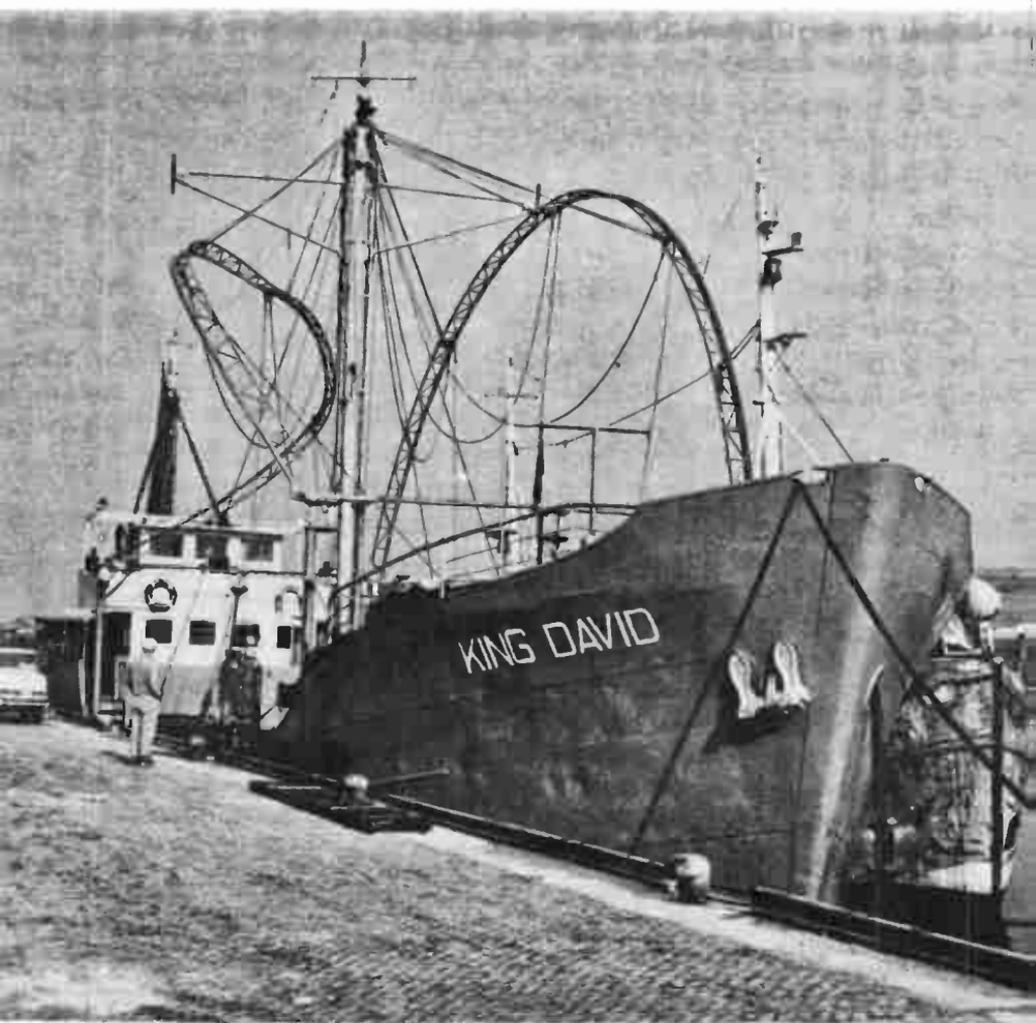
*The Capital Radio ship back in Ijmuiden Harbour with a hopelessly twisted antenna damaged during the lowering operation at sea.*
