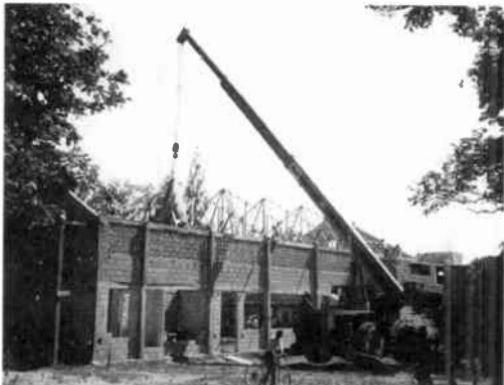
The borrowed crane hoists the steel trusses into place
