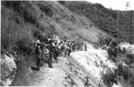
The initial work on the road to Du Pin was done by hand in 1982
