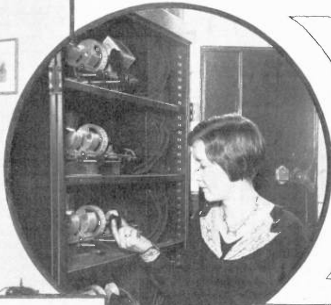
New Wrinkle in Radio for Hotels—This picture shows how Mrs. Belle Barnett turns on switch in apartment in Canterbury Court that operates a loud speaker. She has five stations at her command. Any apartment may play any of the five stations at any time without cross-talk. The master set seen in radio room off lobby. Also Mrs. Carroll Pyne.
