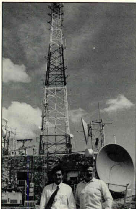
Ricardo Castillo, Vice President of Operations, shown with David Stewart, Chief Engineer at KBNA AM/FM, at the FM transmitter site on the top of Franklin Mountain Range, El Paso, Texas.
