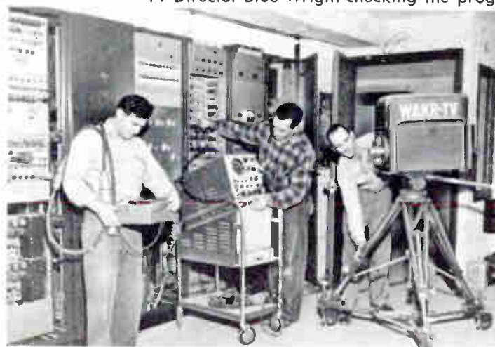
Checking the control room and studio equipment at the Television Center's master control room are (left to right) engineers Jess Nemeth, Chick Girt and Ed Whitlock.
