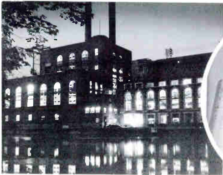
The Gorge power plant of Ohio Edison Company, located on the Cuyahoga River in Akron.
