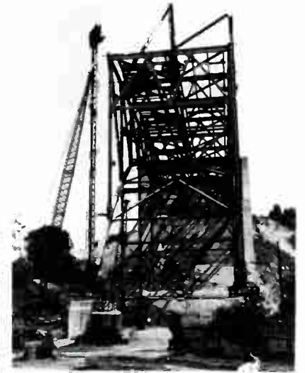
Expressway Bridge under construction.
