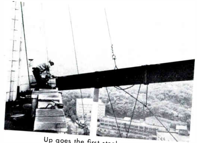
Up goes the first steel support.
