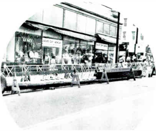
Steel framework on Mill Street for WAKR-TV tower.
