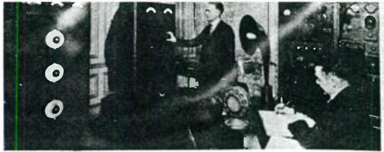
2 EARLY TRANSMITTER: The first WFI broadcasts came from the Strawbridge and Clothier Store . . . those of WLIT, from Lit Brothers. Together they became WFIL in 1935. ED DARLINGTON and DICK DELP were among WFI's first engineers. Both are with WFIL today.
