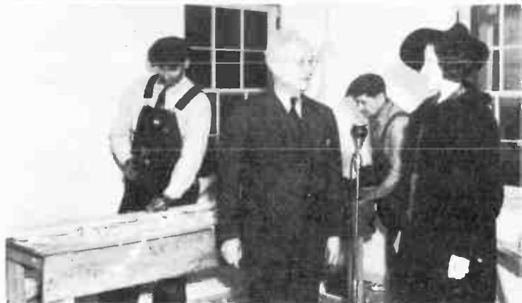
Above—Throughout construction of "Radio's Model Home" being built in downtown Cleveland by the Cleveland Low Cost Housing Association, each step has been relayed to WGAR listeners. In the photo are: Miss Muriele Reid of the Builders' Exchange and Mr. R. L. Hawkins of the Cleveland Paint, Varnish and Lacquer Association during a broadcast interview.
