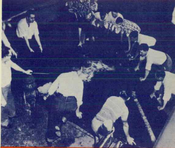
Making a catchall for drafting water in emergencies using a salvage cover. Auxiliary Firemen Trainers at Engine House No. 42. Captain Elmer Ludwig in background at right.
