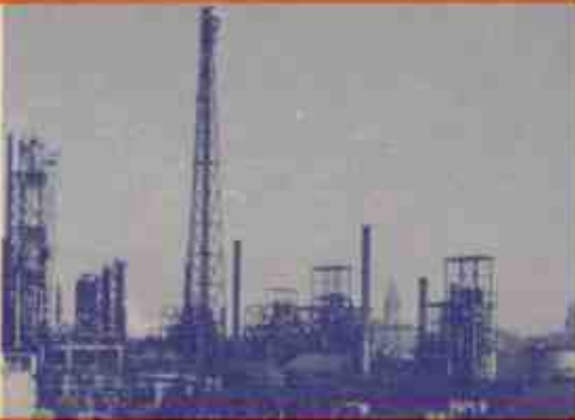
One of the tallest industrial structures in Ohio, is the new Cat Cracker at the No. 1 Refinery of the Standard Oil Co. in Cleveland (John Trauger - Standard Oil Co. Ohio)
