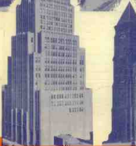
The Ohio Bell Telephone Building in downtown Cleveland is a carefully guarded communications center. (Ohio Bell Telephone Co. Photo)
