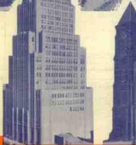
The Ohio Bell Telephone Building in downtown Cleveland is a carefully guarded communications center. (Ohio Bell Telephone Co. Photo)
