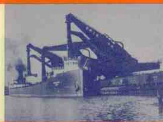
In ore receipts Cleveland leads all lower lake ports with 15 million gross tons in a busy year. Here the Erie Railroad's gigantic Hulett unloader is removing 17 tons of ore from a ship's hold on each trip. (Erie Railroad Photo)
