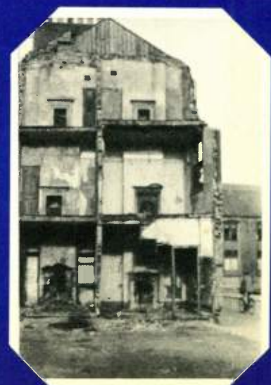
All that's left of a once comfortable tenement house.
