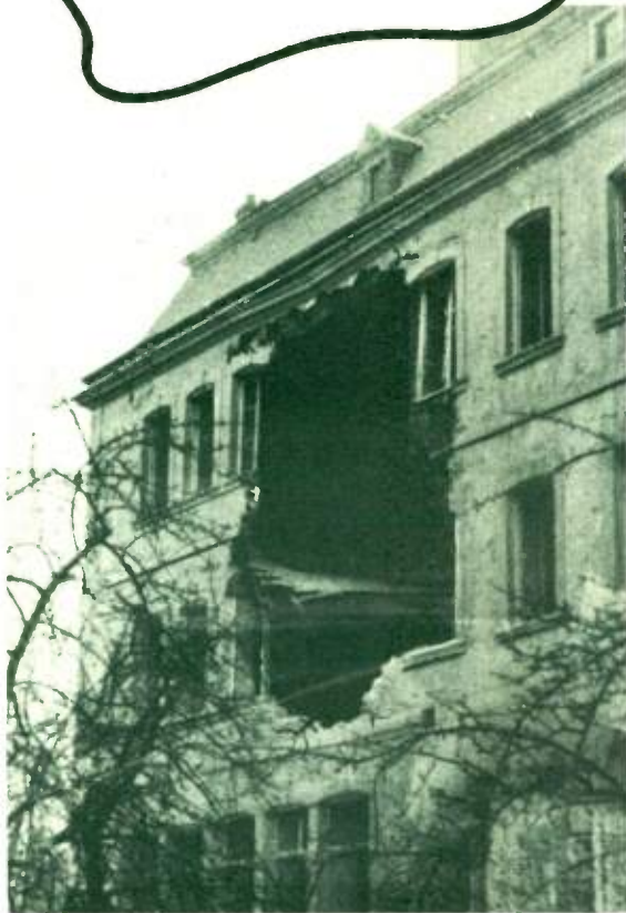
Shell riddled building adjacent to Luxembourg Ministry of Agriculture. Herb was billeted next door while 16 shells fell around the structure.
