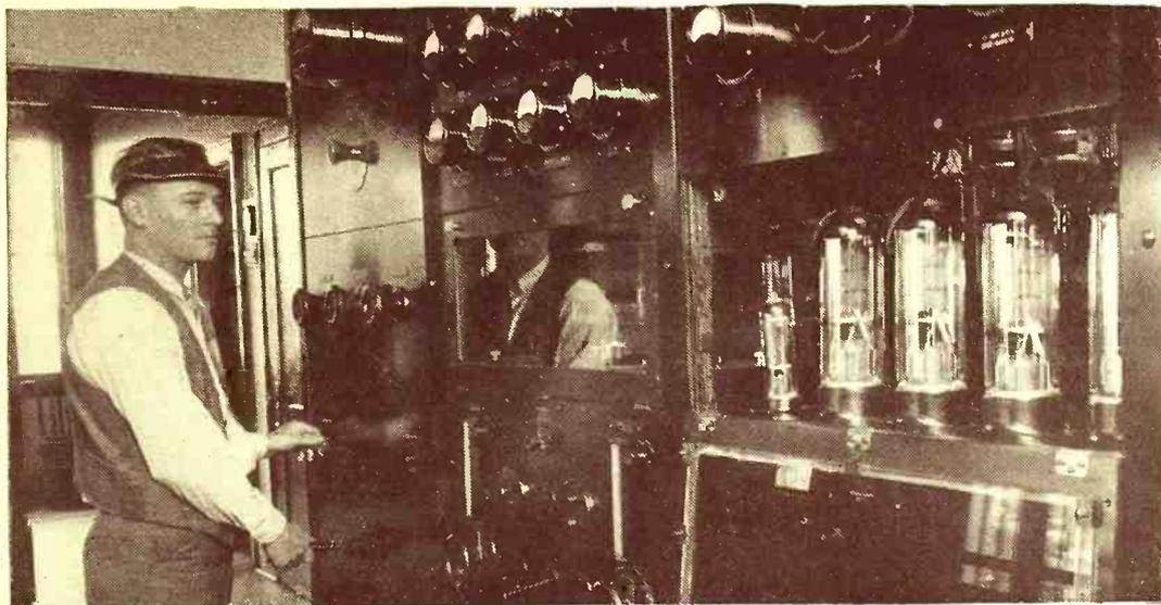
At the left is Homer Courchene in the act of throwing in the switch after the tubes have been heated up to the proper temperature so that you may receive the many programs that go out over WLS every day of the year. A total of 17,000 volts of electric current pass through the rectifier tubes and are here changed from alternating current into 10,000 volts of direct current.
