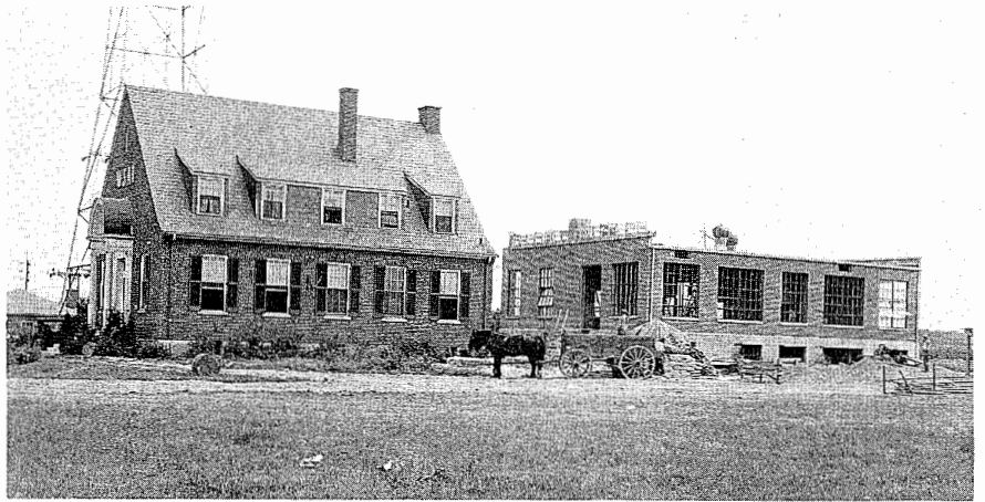
View from North of the facility. This building was to eventually have the rear wall knocked out to contain the 500 KW monster. This construction took place in 1928 to house the 1927 Western Electric 50 KW rig.
