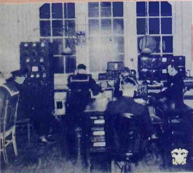
Some of the delicate radio equipment in a Navy radio room.
