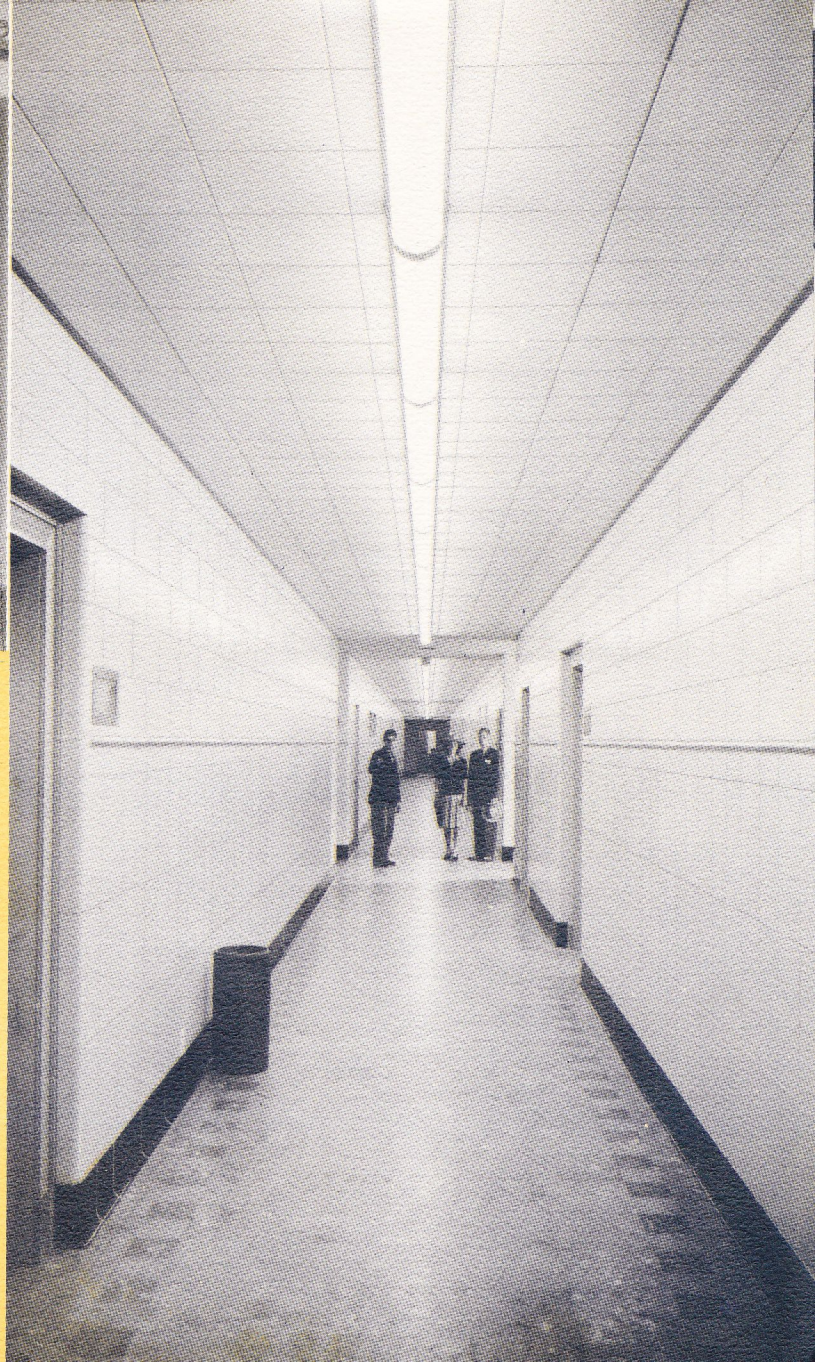
Tile walls and floors and special lighting keep the corridors at Radio City bright and clean.
