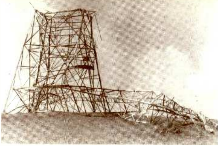
After the winds! The WWVA 225 foot transmitters lie crumpled on the ground at the West Liberty transmitter site, destroyed by 100 mph winds on July 28, 1936.
