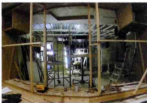
6. Looking into the control room from the studio; showing ceiling mounting for video monitors and the projection screen that retracts into the ceiling. Main monitor speakers are free-standing. (Week 13)
