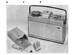
PHILIPS have extended their range of tape recorders with the Philips Starmaker. Among the features of this new machine, is a vertically styled cabinet designed to take a large (6½ in. diameter) loudspeaker for quality sound reproduction.
