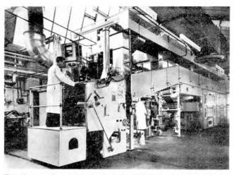
Fig. 19: A modern coating machine about 50 ft. long, weighing 16 tons. Roughly three-quarters of the weight and volume consists of air filtering and conditioning equipment. The precision coating head, at near end, is under the close supervision of a skilled operator, here shown controlling a "dry" practice run. Speed of coating: 200 ft. per minute on to a foil 15 in. wide and up to 7,500 ft. long. (Photo by permission of M.S.S. Recording Co. Ltd.)
