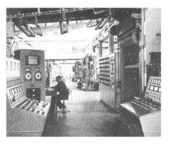
The beginning of the line. Luvitherm film is rolled from heated plastic grains and routed overhead to stretching equipment.
