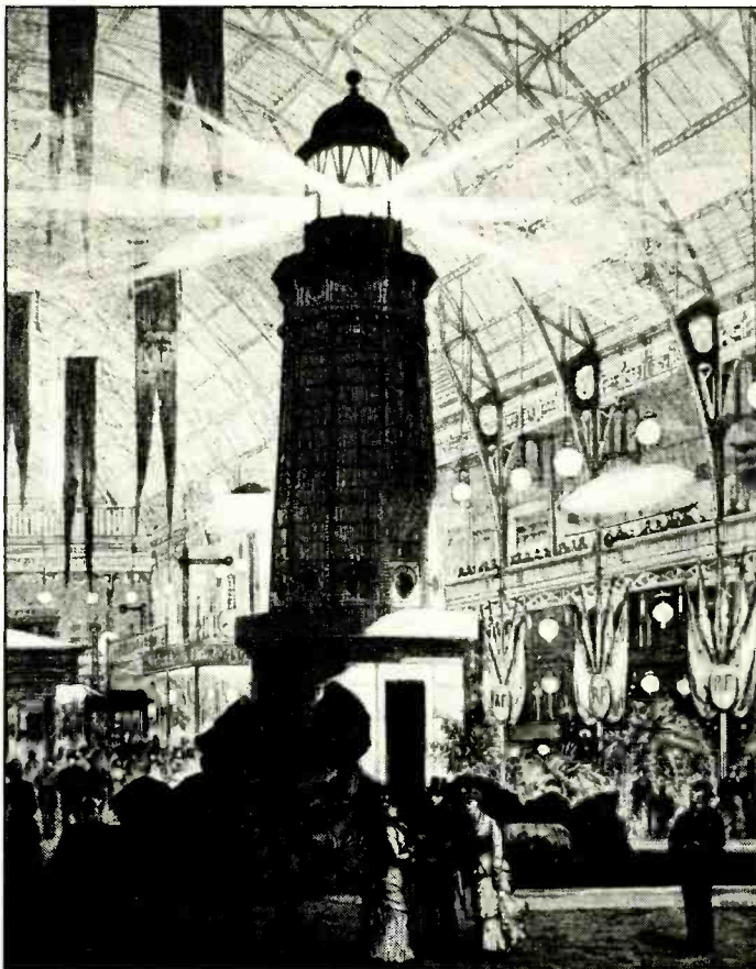
An electric lighthouse, fitted with Fresnel's lenses, was a centrepiece of the Exhibition in 1881
