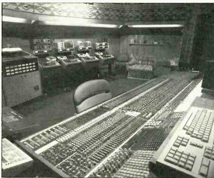
Control Room A
