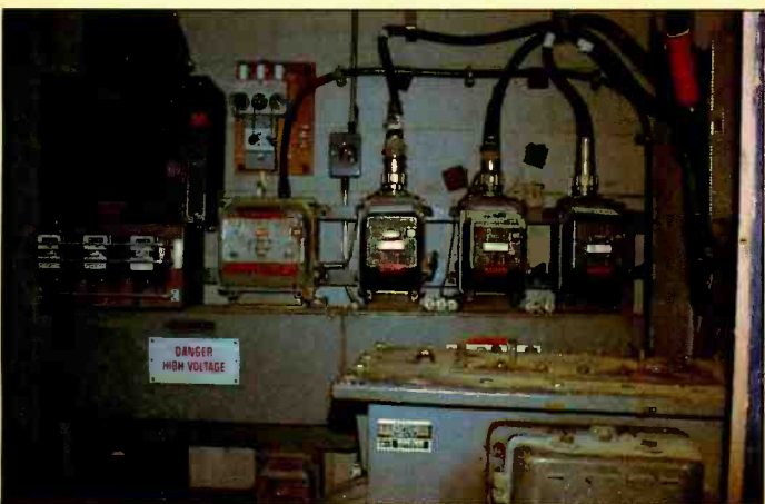
Don't blame us—blame these. Loss of sound due to blown 500 A fuse
