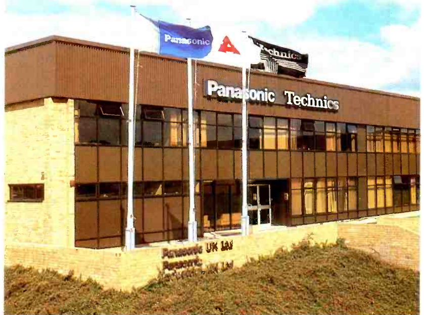
Headquarters of Panasonic UK Limited
